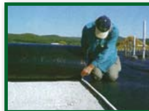
2. Seal using NOFP's patented self-taped seams
